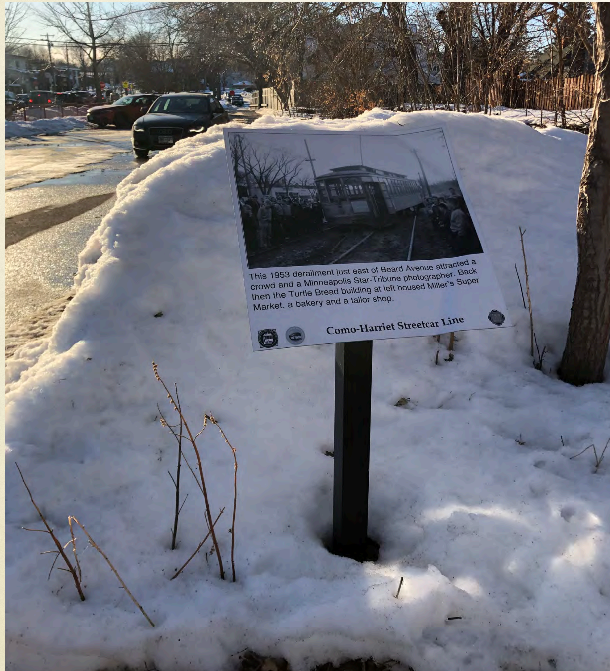
Mounted at a 45 degree angle on square steel channel posts set in concrete
